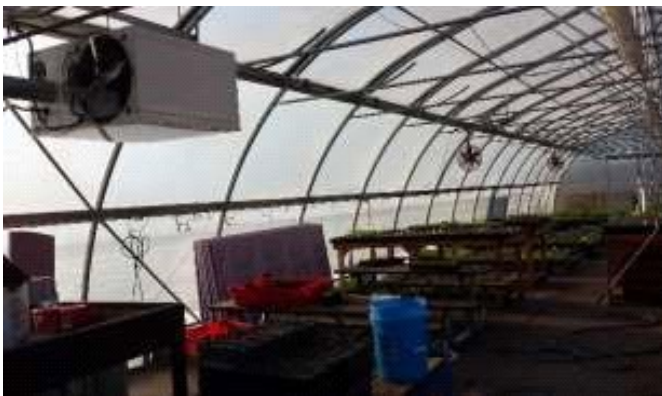
Figure 2. Interior View of the Greenhouse
