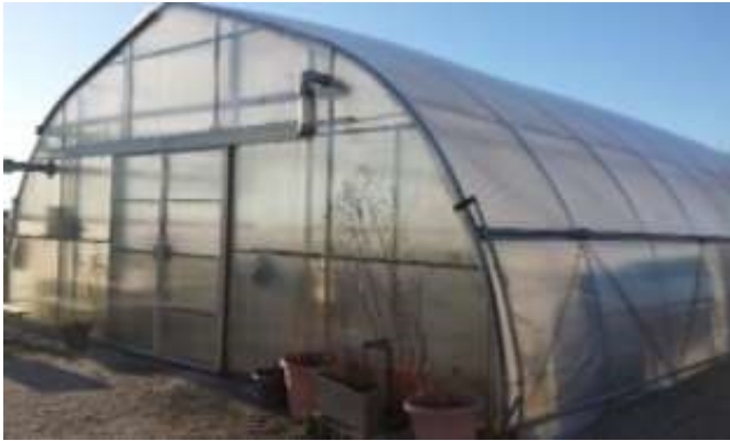
Figure 1. Exterior View of the Greenhouse
